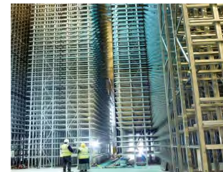
High density storage, Building 31
